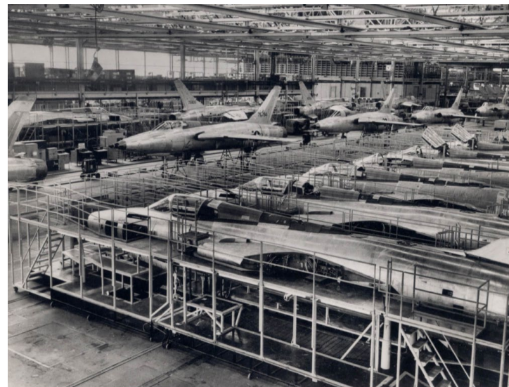
Republic F-105 production plant, Hagerstown, MD
