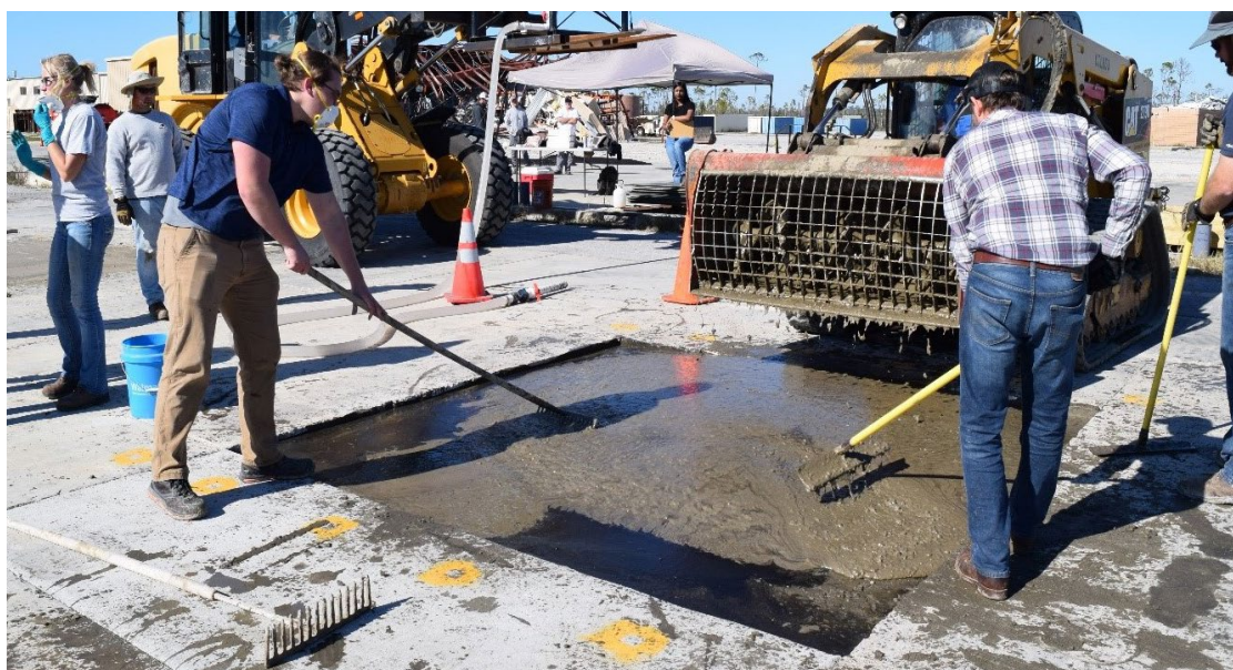
Figure 6: Innovative repair materials developed to use locally available material
