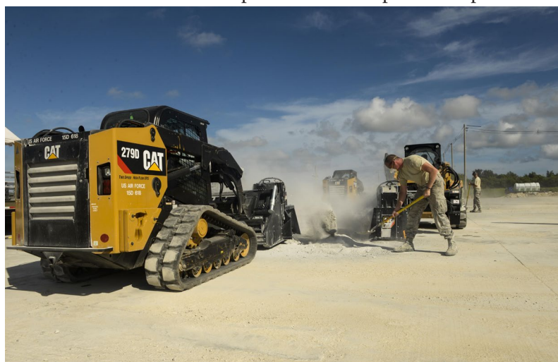
Figure 5: Airmen practice airfield damage repair
